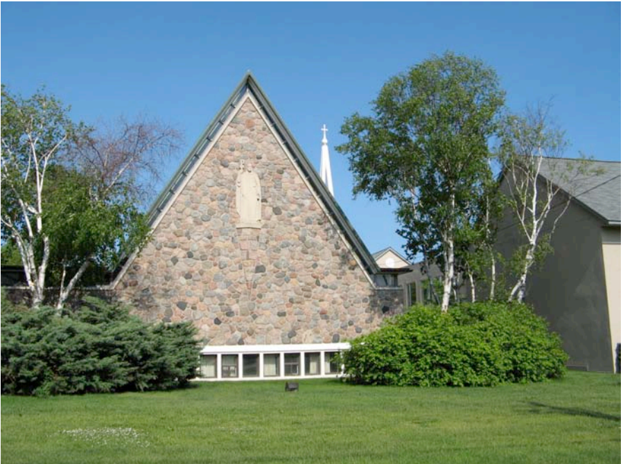
Oriole-York Mills United Church, Front View
